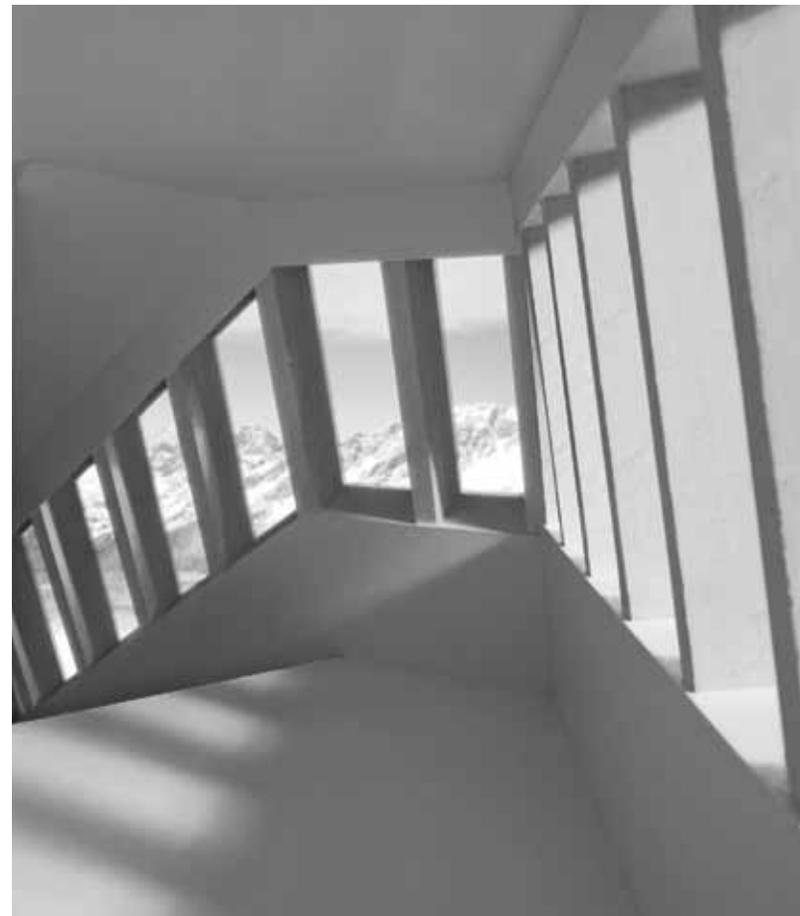
Ribbon windows, mirroring the surrounding mountain ridge and angled staircase, stream light into the hut and enhance thermal energy.
