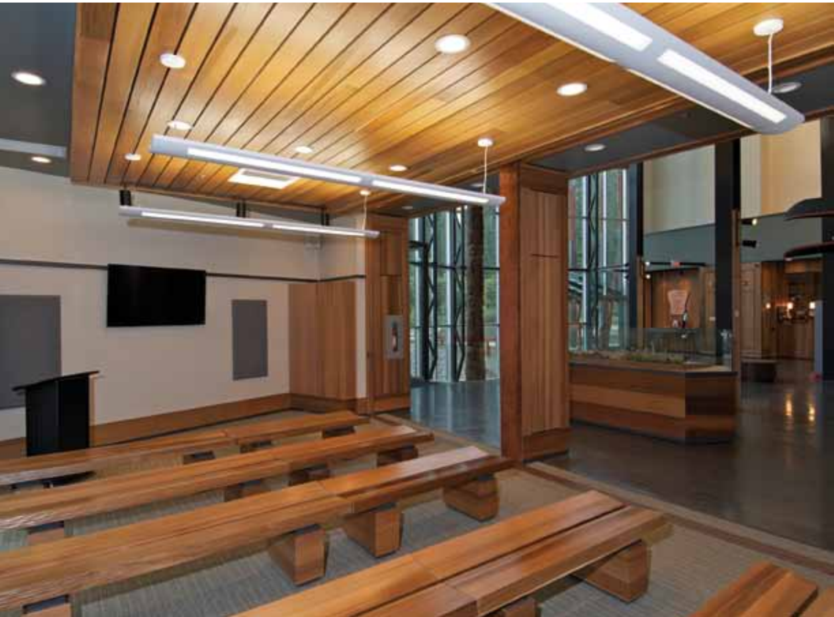
The museum serves as both a learning center and gathering place. Red and yellow cedar, which are native to the area, were used throughout the building.
