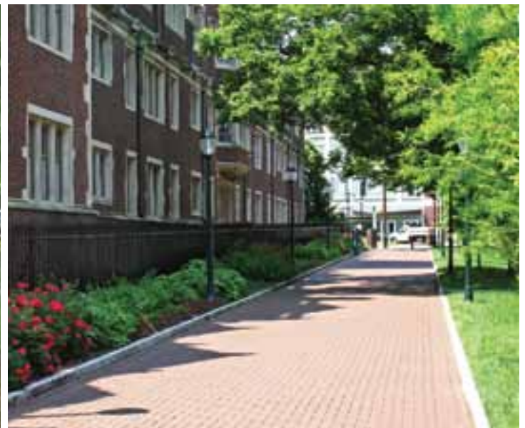
Woodland Walk looking west. The new pedestrian walk paved with unit pavers and edged with new granite curbs. A new lower fence is set back to allow for planting beds that edge the walk. New light standards also edge the walk on both sides.
