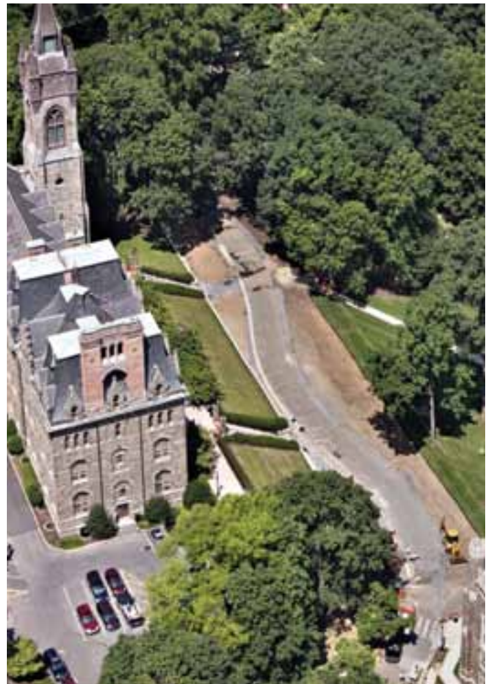
Aerial view of Library Drive Walkway under construction.
